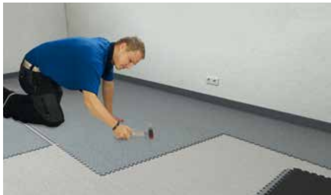
Tip: Laying with a soft-face hammer
